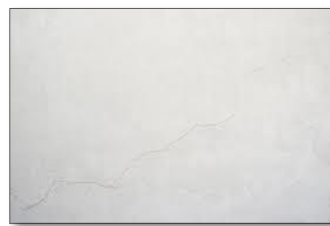
Hairline Cracks
